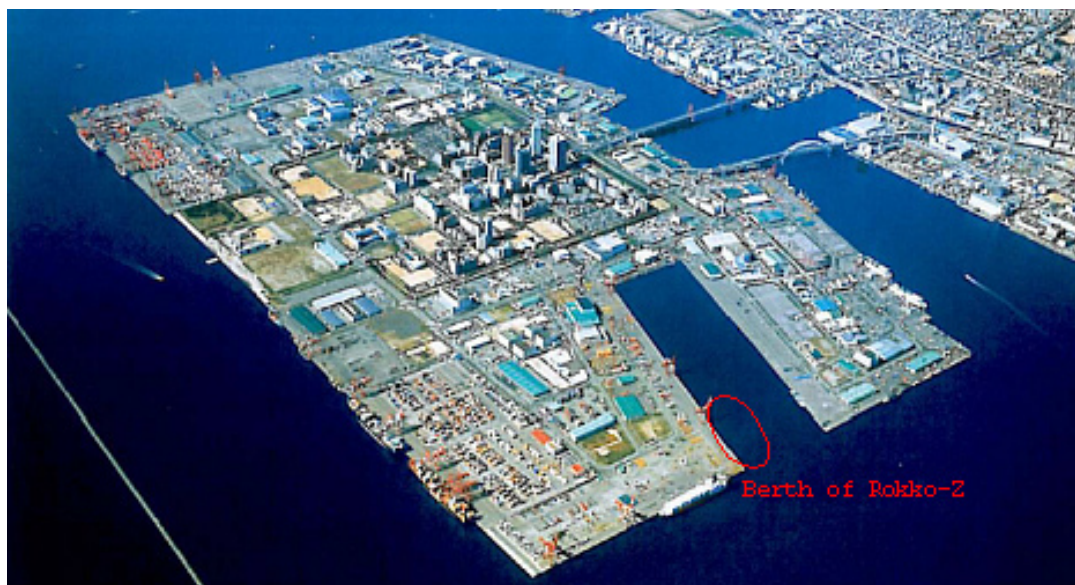
Aerial view of the location of Rokko-Z berth in Kobe.
