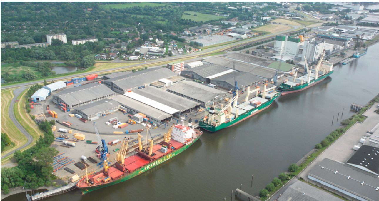
Aerial view of Wallmann & Co. (Photo © Wallmann)
